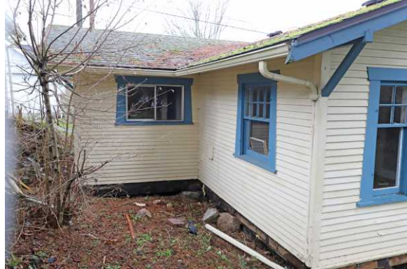
South facade, looking west.
