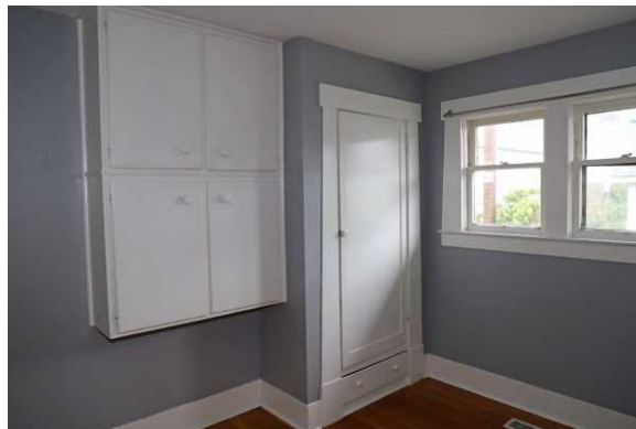
Central bedroom, looking southwest.
