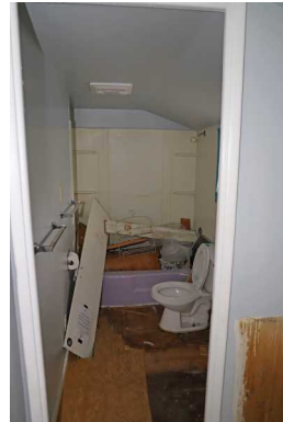
Bathroom, looking west.
