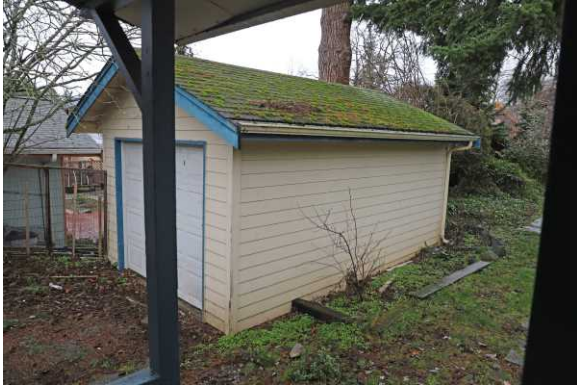
Porch, looking northeast.
