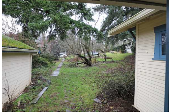
Porch, looking east.
