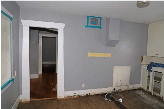
Kitchen, looking southwest.
