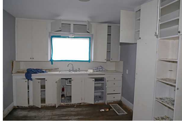
Kitchen, looking west.
